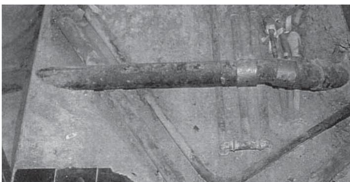
Water and waste water conduits that are embedded in concrete violate the principle of separating components of different life expectancies.
